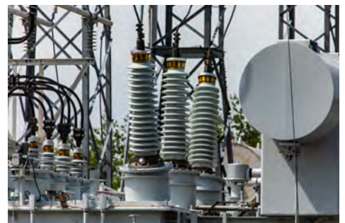
▲ Alumina, an example of an advanced ceramic, is commonly used as an insulator to hold high-voltage electrical transmission wires.
