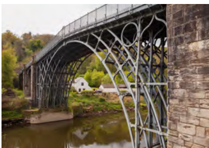
▲ Cast iron: an iron-carbon alloy and popular structural material because of its low cost
